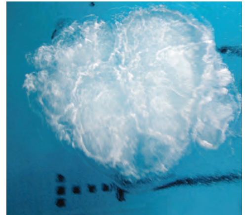
Embedded Pool Floor Air Diffuser
